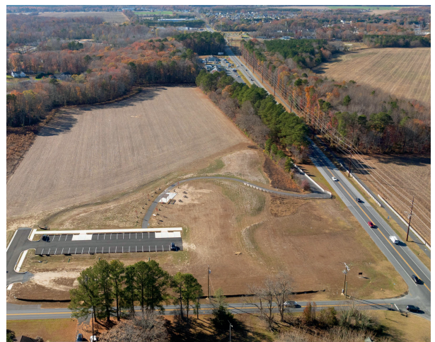
AERIAL LOOKING WEST, NEW ASPHALT PARKING AREA AND TRAIL CONNECTION TO LEWES TO GEORGETOWN BIKE TRAIL
