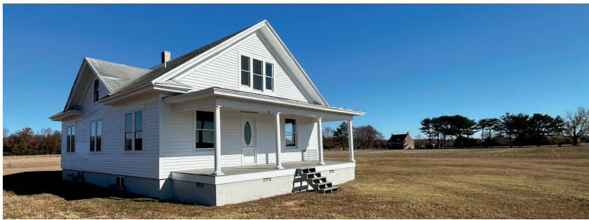
WILLIAMS-LITCHFORD HOUSE RELOCATED TO THE WEST SIDE OF ICKFORD PARK, CANNON-MASTON HOUSE IN THE BACKGROUND
