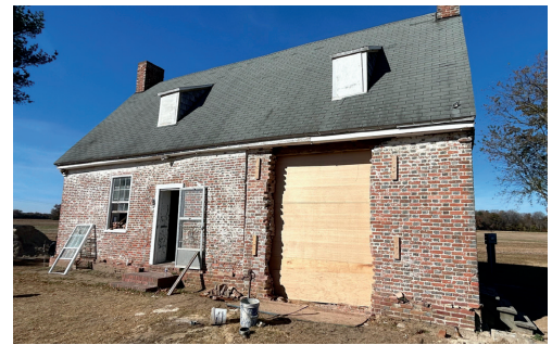
CANNON-MASTON CONSTRUCTION IN PROGRESS
