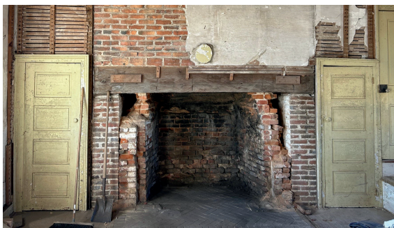
CANNON-MASTON INTERIOR RENOVATIONS
